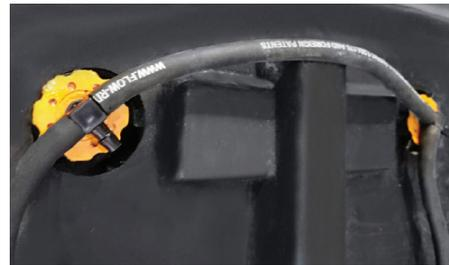
**5.** Connect the water feed line near the center of the battery onto an unused swivel connector port. Refer to the installation diagram for the recommended location.
