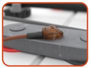
Step 5: Anchor the half voltage lead (brown wire) to an inter-cell connector halfway between the positive and negative posts. Coat all anchored hardware with supplied no-ox grease.
